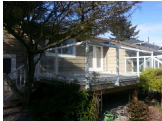
After: white aluminum glass railing
